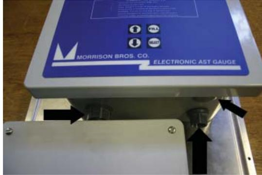
*Above:* This picture shows the conduit fittings used for wiring the console. The vertical arrow on the right shows where the conduit for AC power will run to. The arrow on the left shows where the barrier connects to the console (factory installed), and the right most arrow shows the 1/2" hole seal that should be replaced with a 1/2" conduit fitting if a PC connection will be installed.
