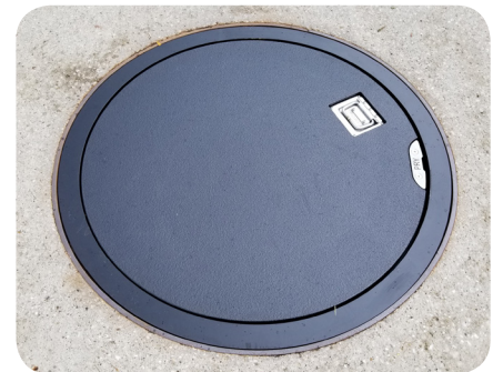
Field installation photo
